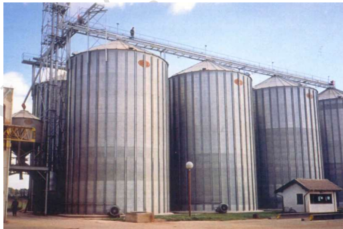
Figure D.22 - Tower storage silo
